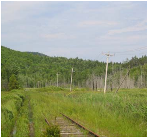
A view of Bangor Hydro's aging Line #13. The proposed Downeast Reliability Project seeks to improve the reliability standards of transmission lines servicing the Downeast region, and will utilize this same corridor.
